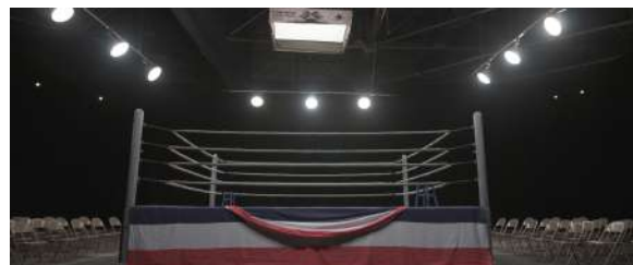
One of the designs, in the center a light box with three Skypanel60 and silk. On the sides, ceiling lights with 1000w tungsten lamps with diffusion and dimmer it
